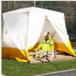
Welding tent/shelter and ground sheet
